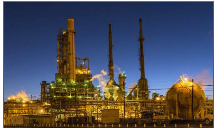
Fig. 8 - External view of a petrochemical plant
