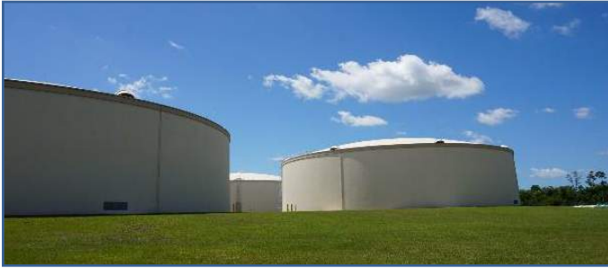
Fig. 2 - Oil storage tanks
